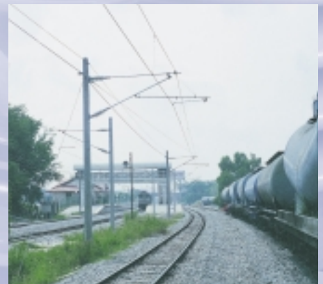
Tension and strut insulators in railway lines
