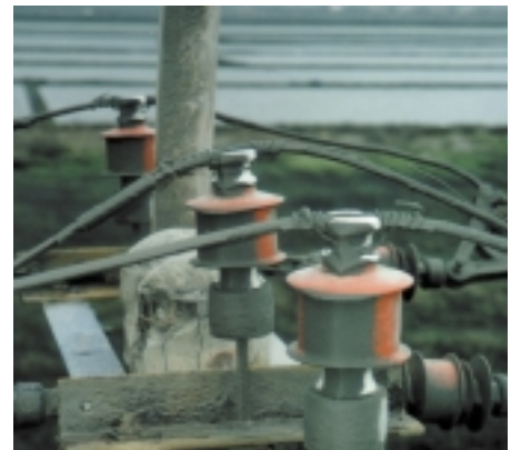
Working conditions of Raybowl insulators
