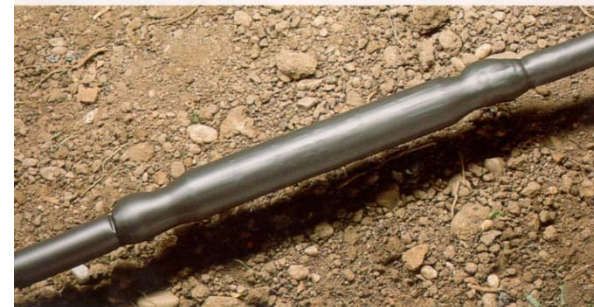
Armoured low voltage cable connection
