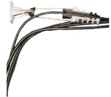
Tension hanger. The conical device tightens and supports the neutral cable
