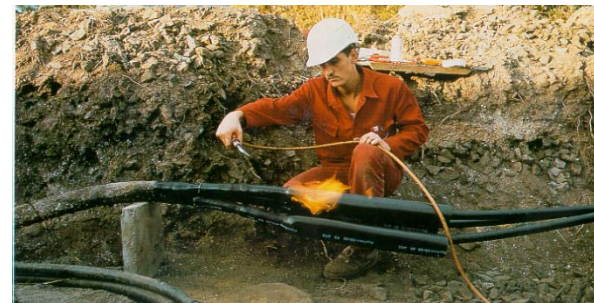
Underground medium voltage connection
