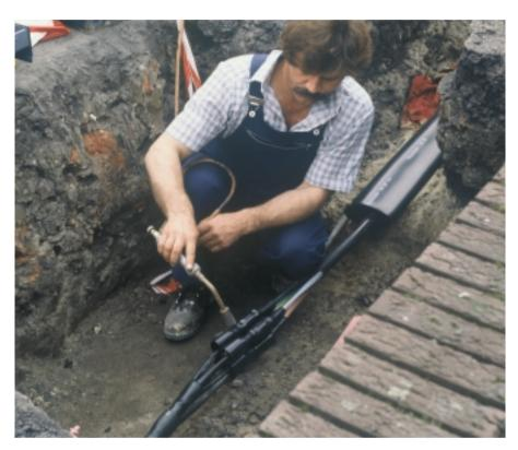
The conductors can be jointed with either mechanical, compression or soldered connectors, which are then insulated by shrinking adhesive-lined thick-walled tubing over them, at the same time finally sealing the cores of both cables.
