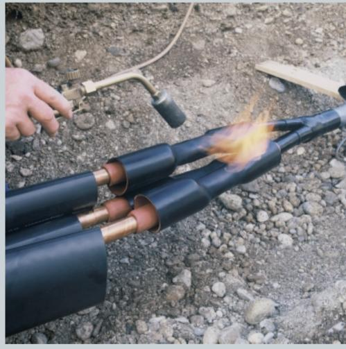
User experience with our system on both paper and polymeric cables has confirmed it as a reliable and efficient technique for jointing plastic insulated cables to existing paper cable networks.
