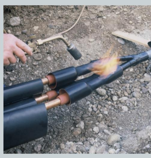
User experience with our system on both paper and polymeric cables has confirmed it as a reliable and efficient technique for jointing plastic insulated cables to existing paper cable networks.
