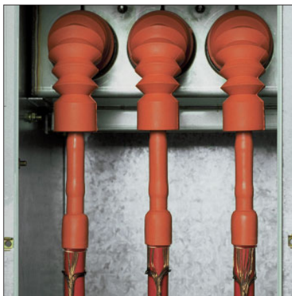
TFTI installed with Raychem bushing boot (RCAB)
