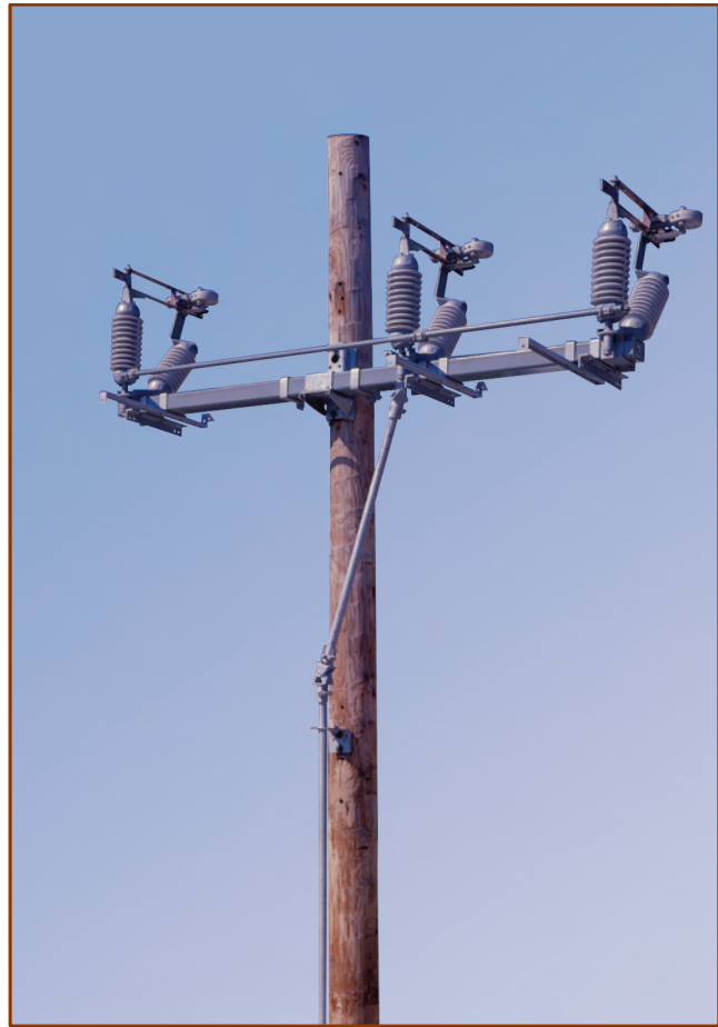
Insulated-base 34.5-kV Side-Break Integer Style Alduti-Rupter Switch.
