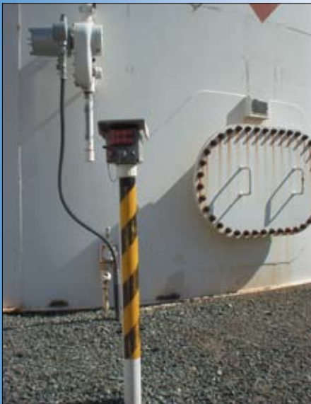
TT5000 Sensor Cable in PVC conduit can be positioned below buried valves or beneath Above-ground Storage Tank bottoms.
