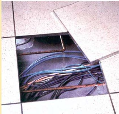
*Placed in the sub-floor of a computer room, the TraceTek system protects your computer equipment by detecting a leak early – and even locating its source.*
