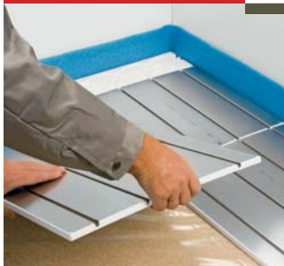
Installation of plates
