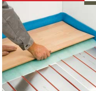
Installation of the wooden floor
