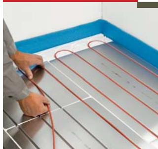
Install heating cable
