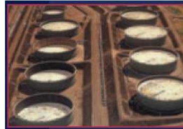
Tank Foundation Heating
