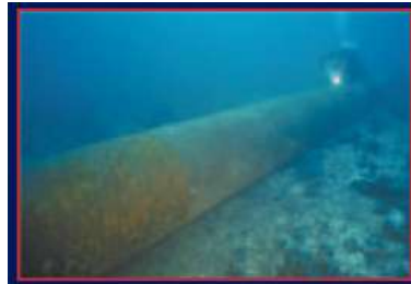
Subsea / Submerged Lines
