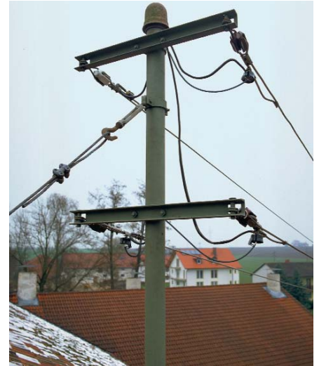
Service entry through overhead system
