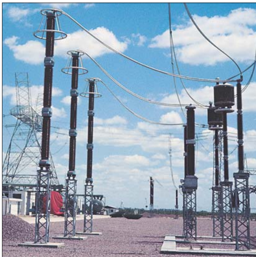
300kV Surge Arresters - Kuwait
