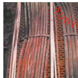
Pyro MI survived in this high rise office complex fire
