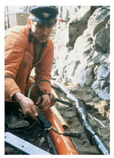
**Ordering information** Raychem joint kits are available for plastic insulated cables with or without armour for up to 1 kV, with 2 to 5 cores and with conductor crosssections up to 300 mm<sup>2</sup>. Joints for larger cross-sections and a full selection table are available on request.
