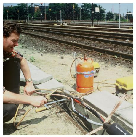
After the conductors have been jointed, the connectors are insulated and moisture sealed out by shrinking Raychem tubing over them. The specialpurpose adhesives are supplied already coated on the insides of the inner and outer joint components.
