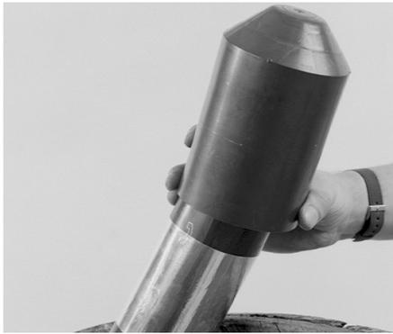
Wipe loose dirt from cable and slip end cap over the cable.
