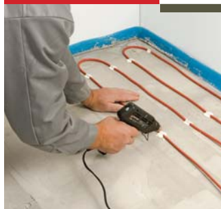
Cable installation
