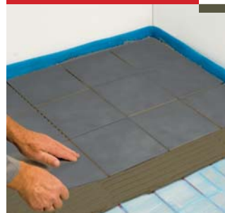
Installation of tiles
