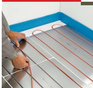
Installation of cable
