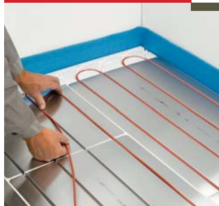
Install heating cable
